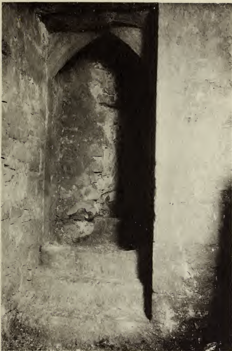
(FIG. 11) VIEW OF DOORWAY FROM ENTRANCE HALL TO INTERIOR OF TOWER, SHOWING LATER ADDITION TO THICKNESS OF WALL
